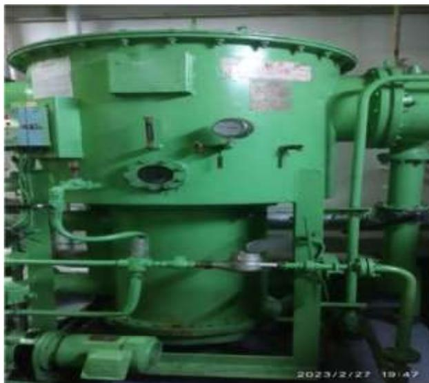
**Gambar 1. Fresh Water Generator(FWG)
